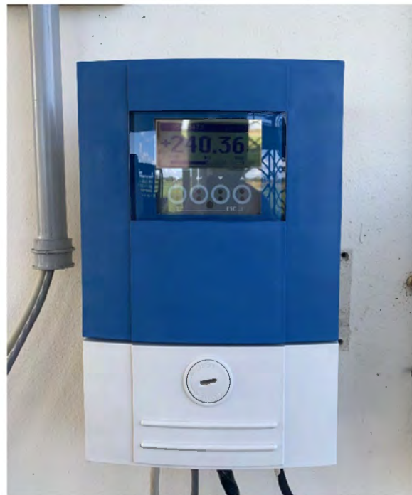
Grit Flow Meter –Transmitter Unit
