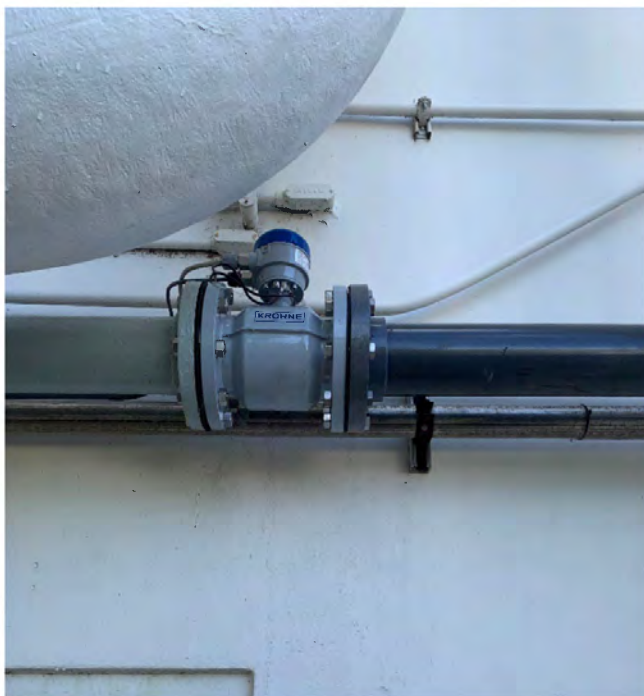
Grit Flow Meter – Inline Magnetic Tube
