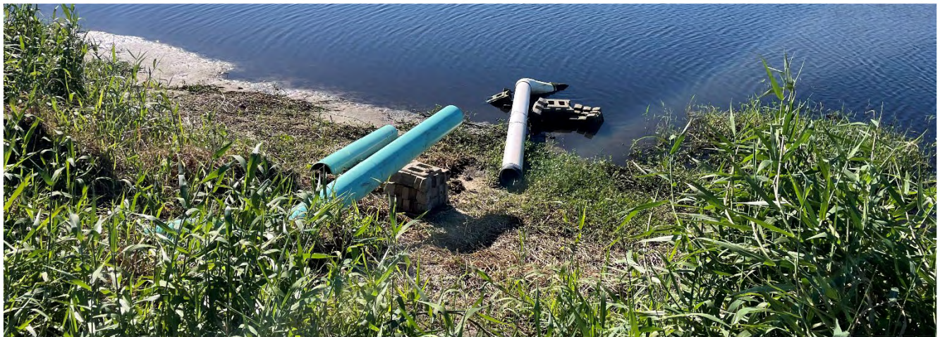
North Canal Pump - Discharge Piping and Support Failure
