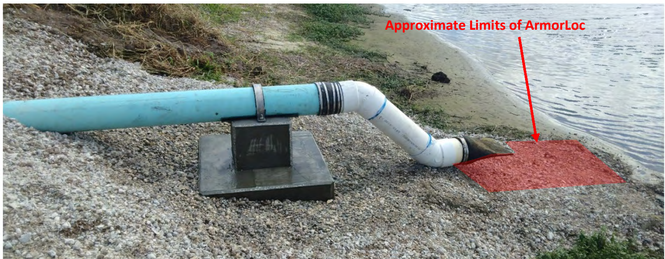
North Canal Pump - Discharge Piping and Support Repair
