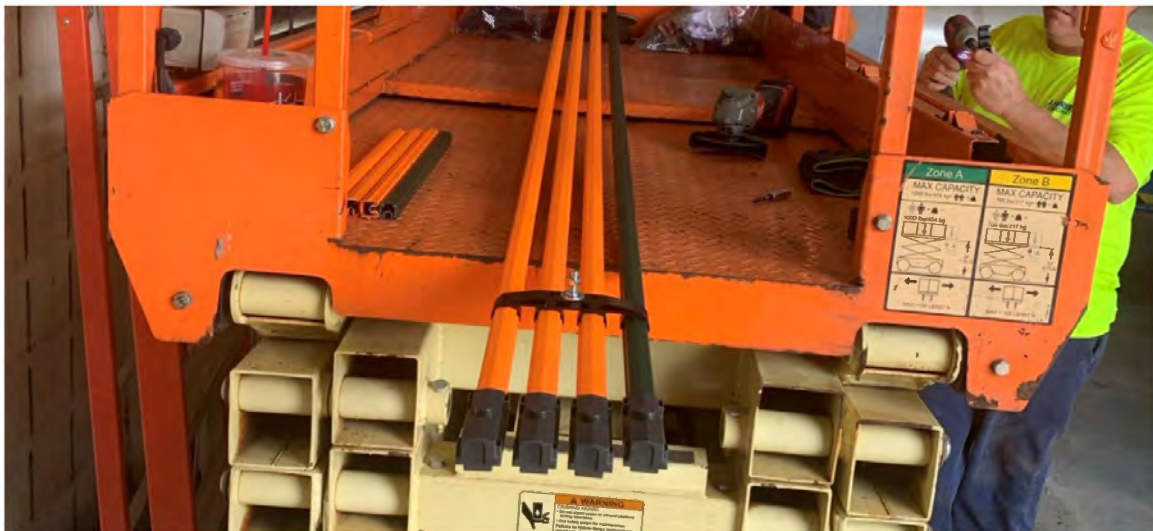
Four (4) Conductor Bar System
