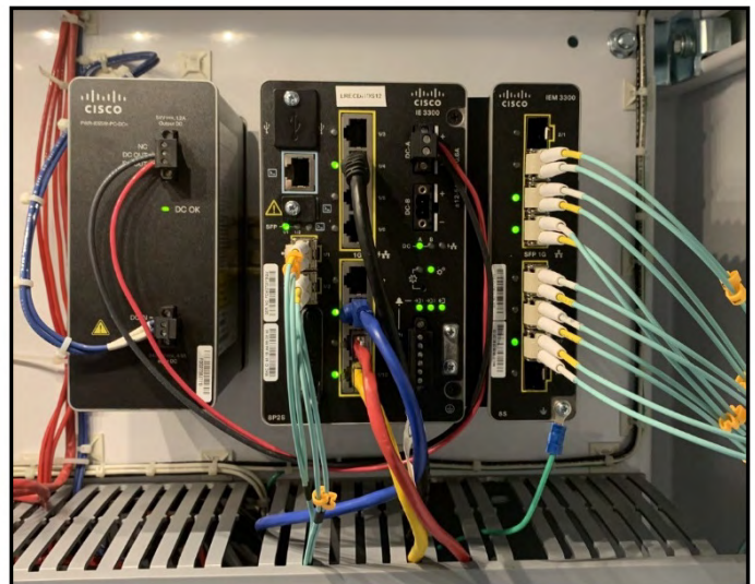
Example Industrial Network Switch that provides connectivity to the industrial control equipment for the treatment plant
