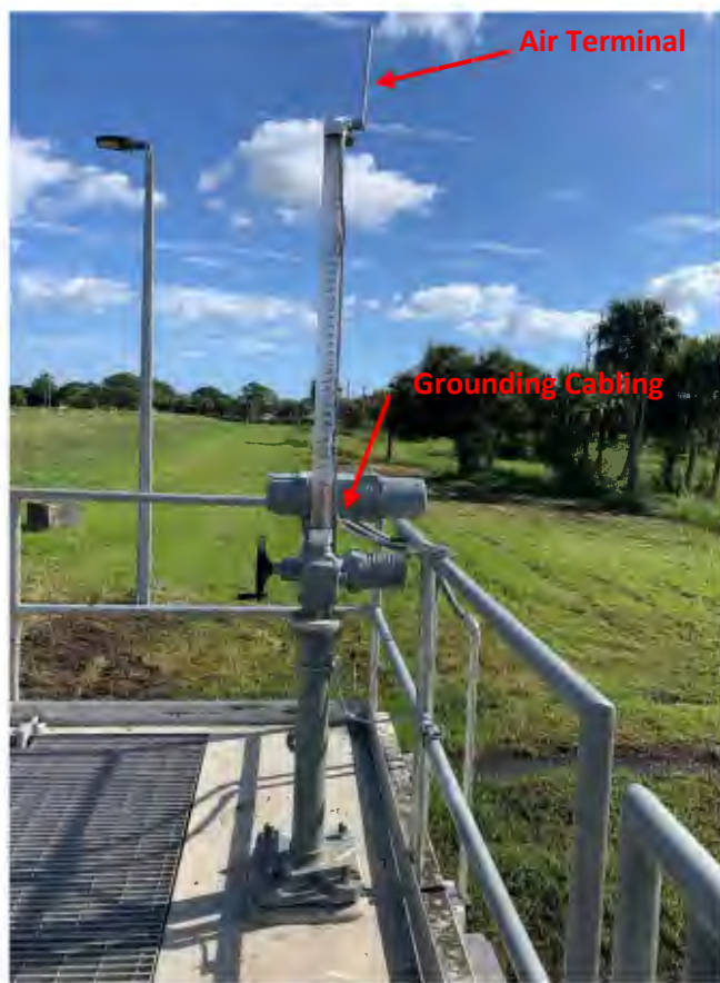
B-Structure Lightning Protection System Improvements
