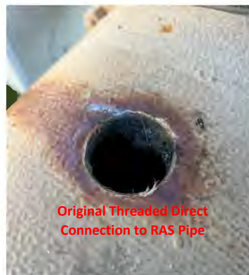
RAS ARV Piping Manifold and Valve Replacement
