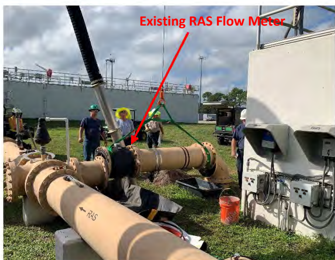
Clarifier No. 3 – RAS Flow Meter Replacement – Pre and Post
