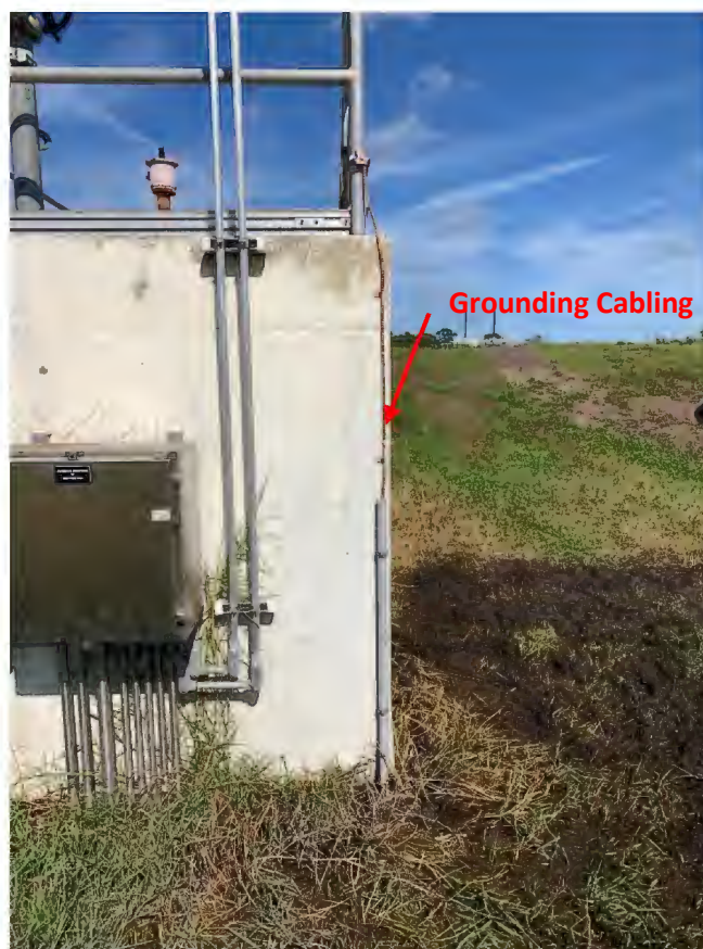
B-Structure Lightning Protection System Improvements
