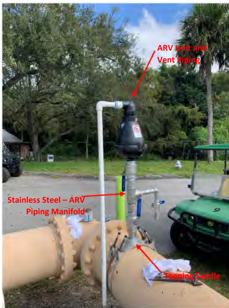
RAS ARV Piping Manifold and Valve Replacement
