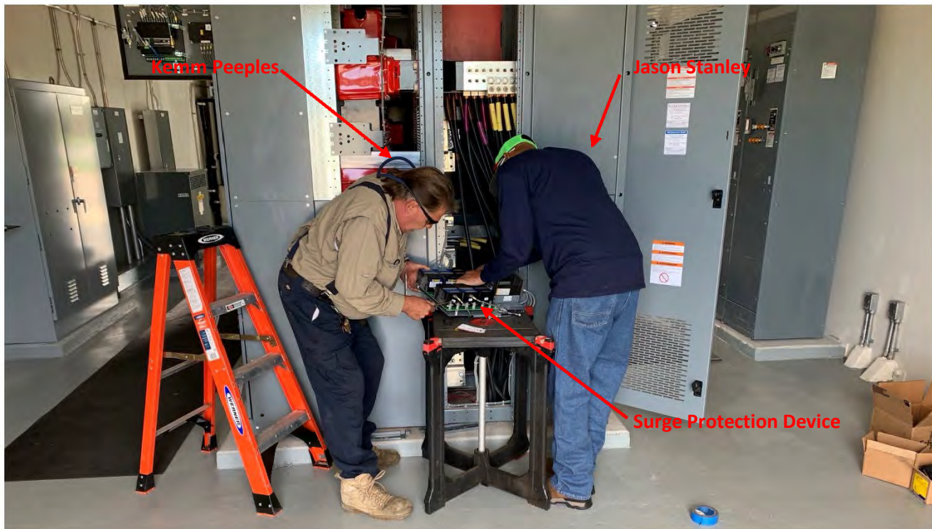
Replacement of ER-13 MDS Surge Protection Device
