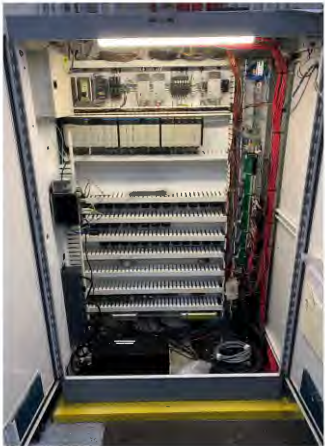
Refurbished Headworks PLC Panel
