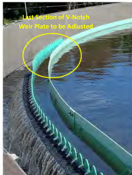
V-Notch Weir Plate Adjustment
