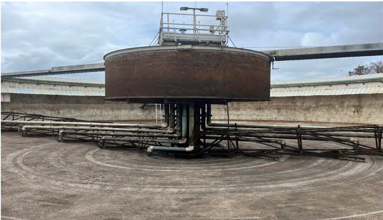
Internal View of Clarifier No. 4
