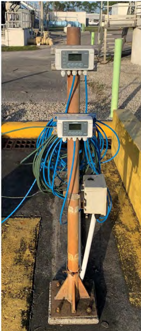
DIW Monitor Level Transmitter Rack
