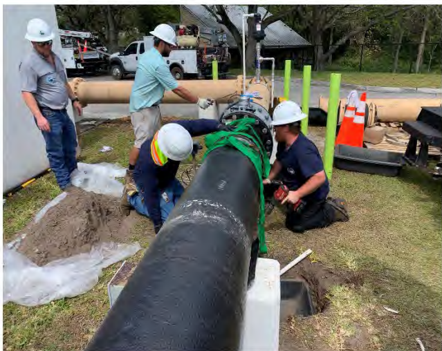
Clarifier No. 4 – RAS Flow Meter Replacement
