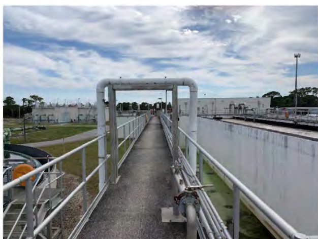
Replaced Schedule 40 PVC Piping
