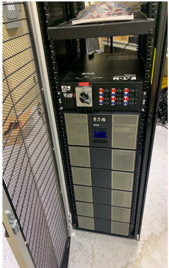
Uninterruptible Power Supply Unit
