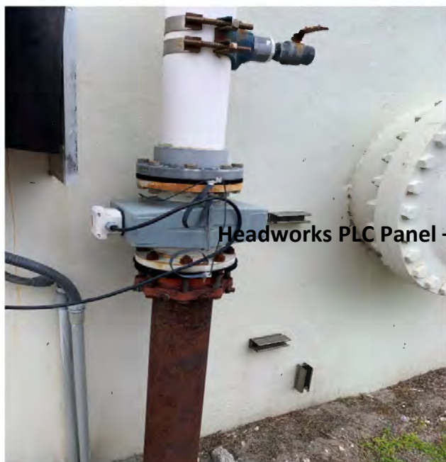
Replaced Magnetic Flow Meter Tube
