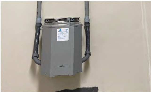
480V to 120V Step-Down Transformer
