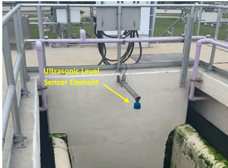
Deep Bed Filter Unit – Ultrasonic Level Sensor
