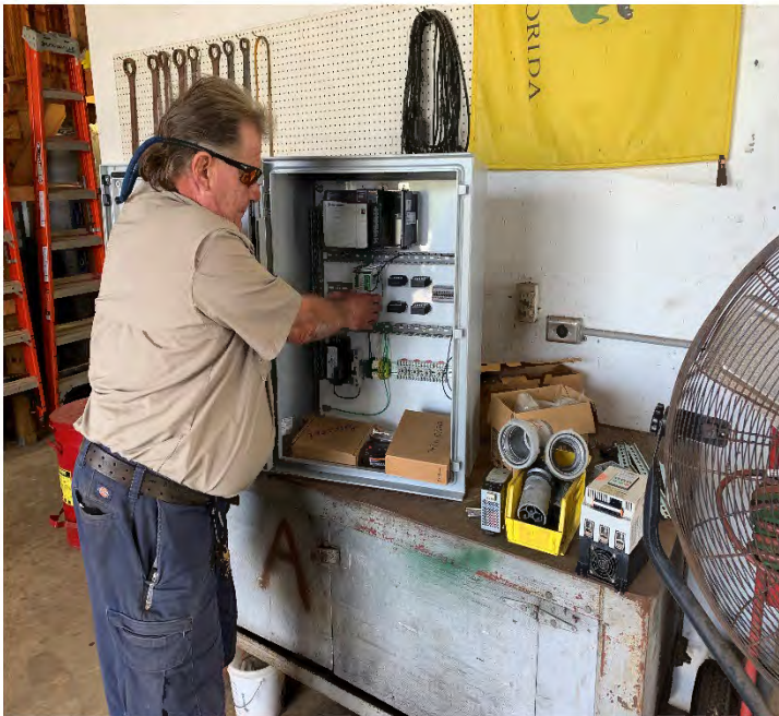
Network Switch Panel Fabrication
