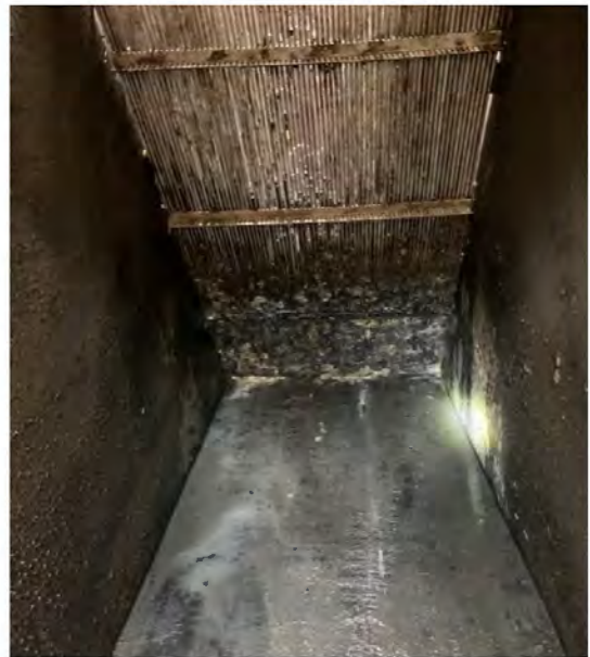
IW Screen Structure – Existing Rack
