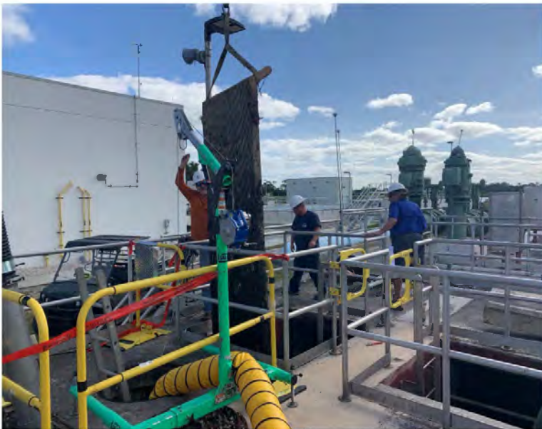
IW Screen Structure – Bar Rack Removal
