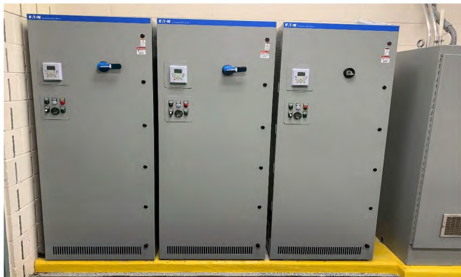
Filter Pump Station No. 2 – Replacement VFD's
