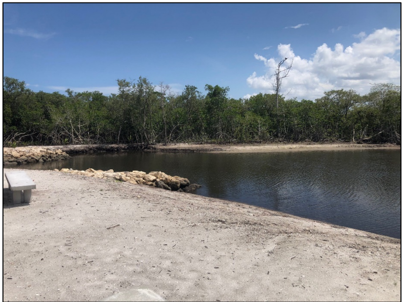
Figure 9. Photo shows recent completion of the interior paddling trails of Sawfish Island. Work was completed just as this assessment was started.
