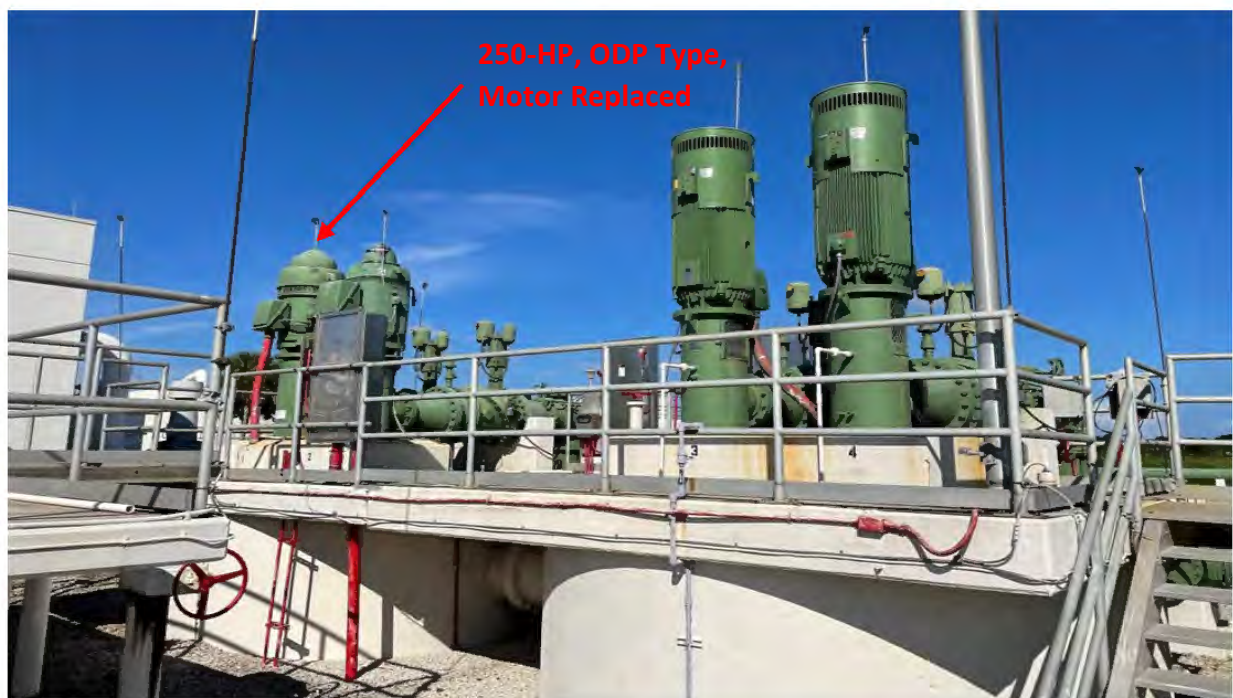
Injection Well Pump No. 2 – Motor Replacement
