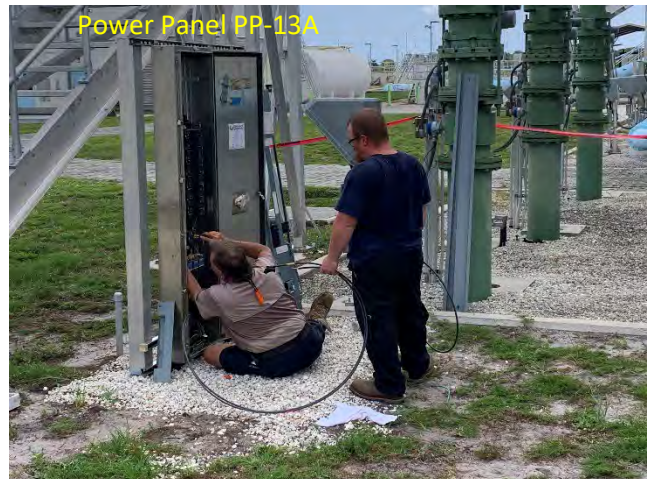
Maintenance Team Members Collaborating to Replace Conductors
