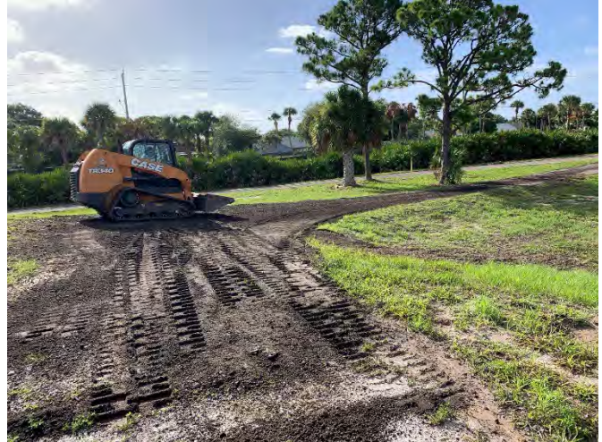
Stabilization Pond Regrade of Earthen Access Road
