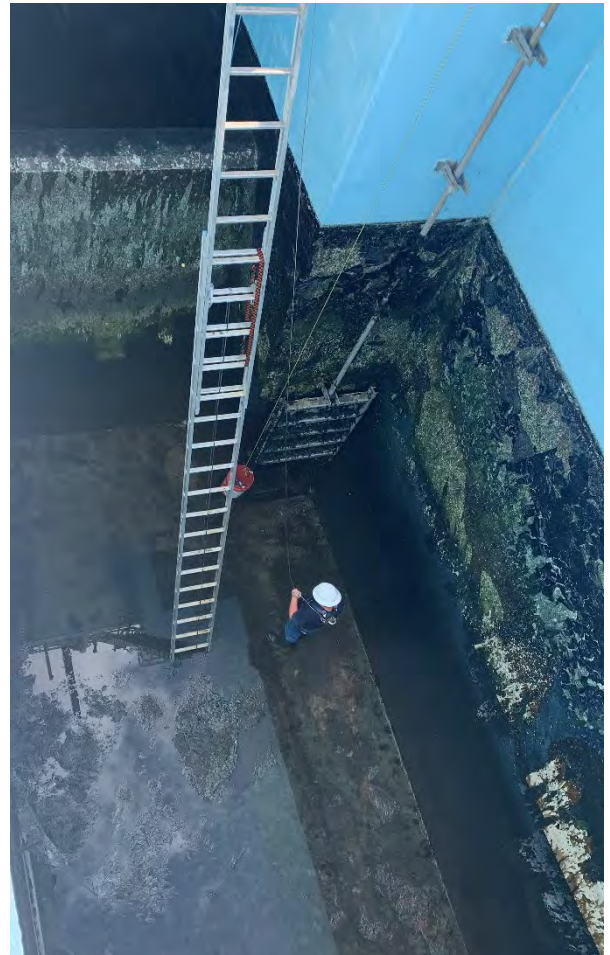
Backwash Storage – Slide Gate Inspection
