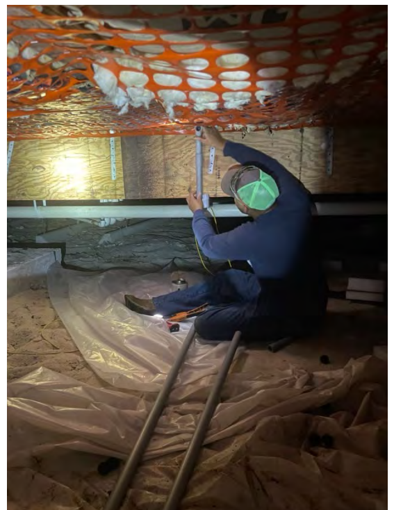
Electrical Work within Crawl Space
