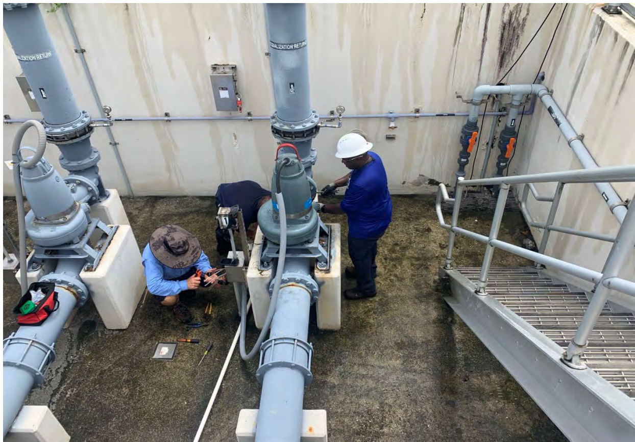
Equalization Pump Station – EQ Return Pump No. 3 Replacement
