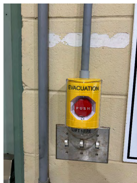
Chlorine Alarm System – Notification System Improvements
