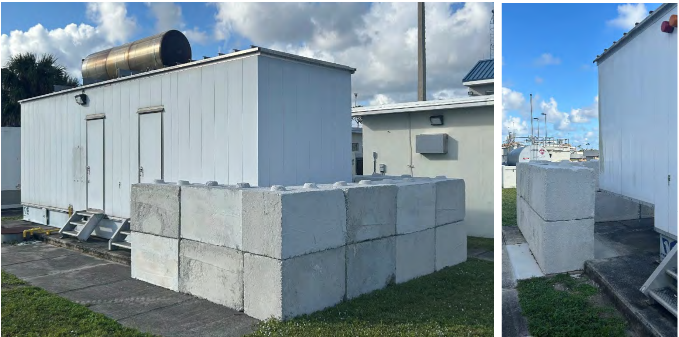
Main Generator No. 1 – Plenum Improvements
