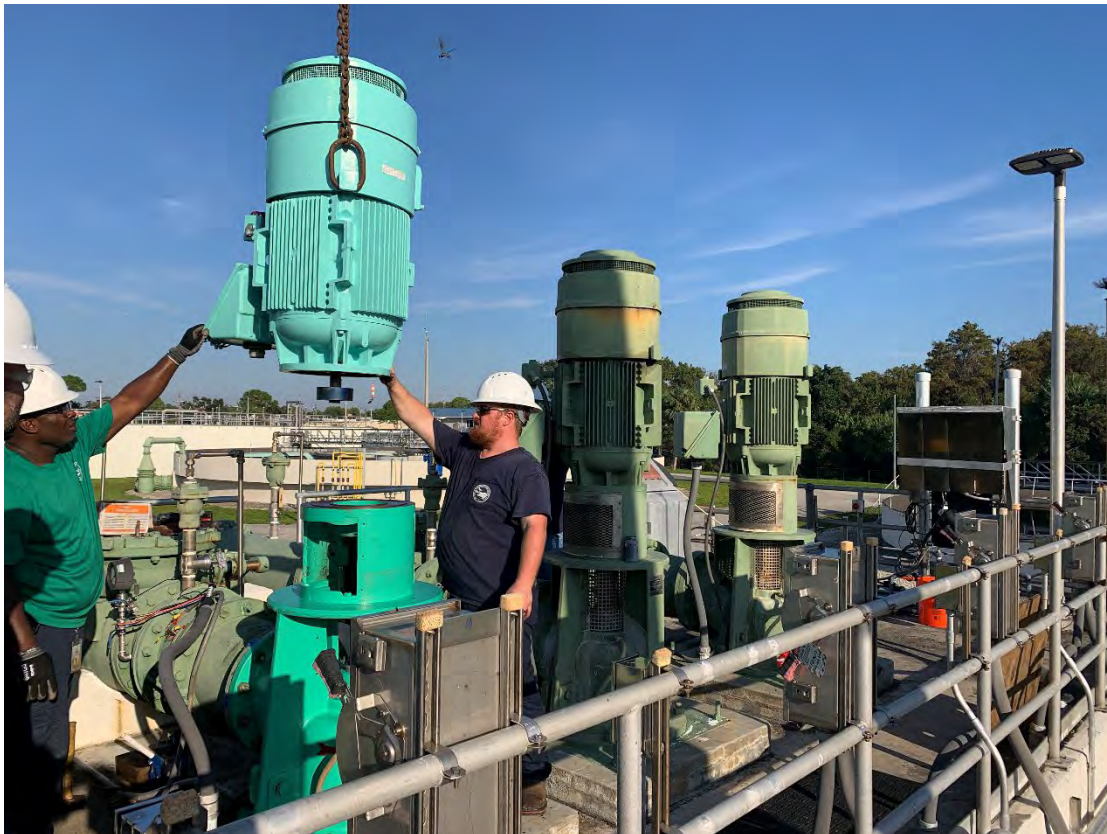
Filter Pump Station No. 1 – Pump No. 3 Reinstallation
