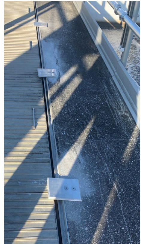
Aeration Basin Structure – Aluminium Cover Stop Plates
