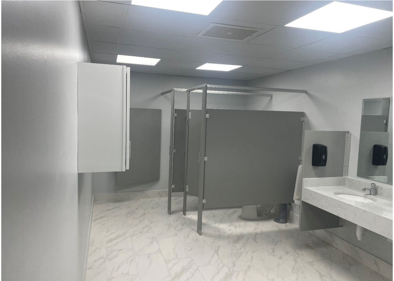
District Administration Building – Bathroom Renovation
