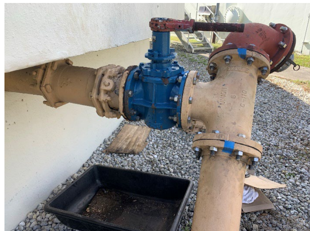
Scum Trough Drain Valve Replacement
