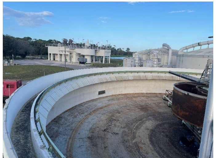
Clarifier No. 4 – Draining and Cleaning
