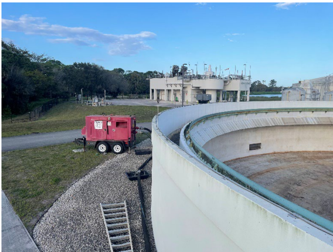
Clarifier No. 4 – Draining and Cleaning
