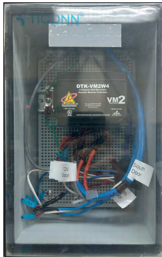
New Surge Protection Enclosure for Door Access Controls
