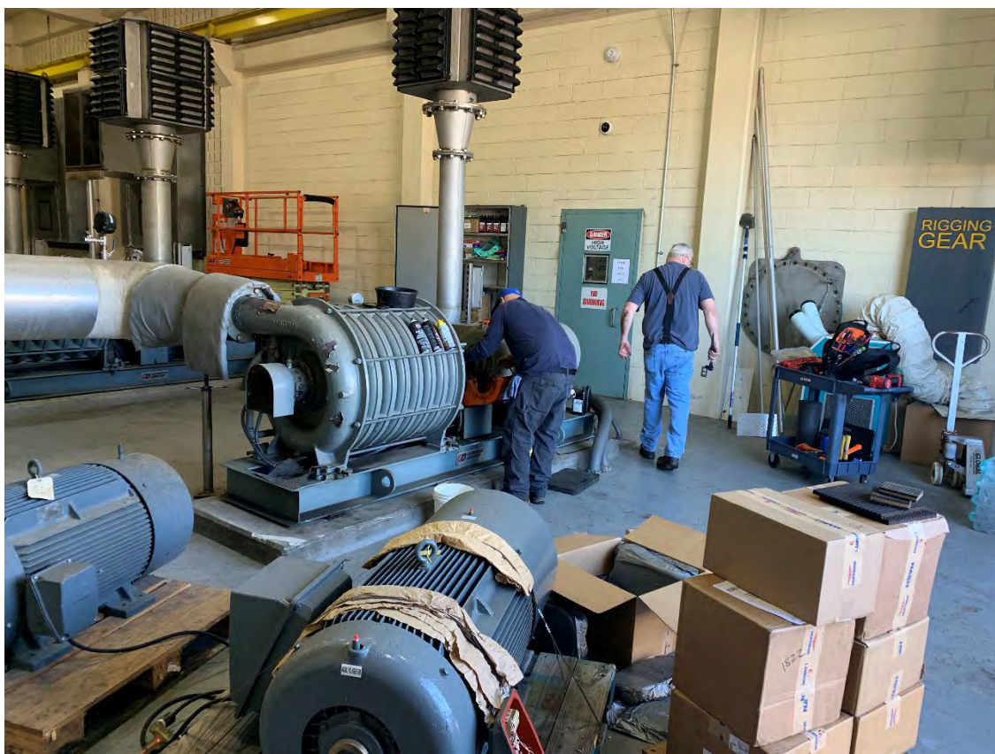
Process Air Blower – Annual Inspection and Maintenance
