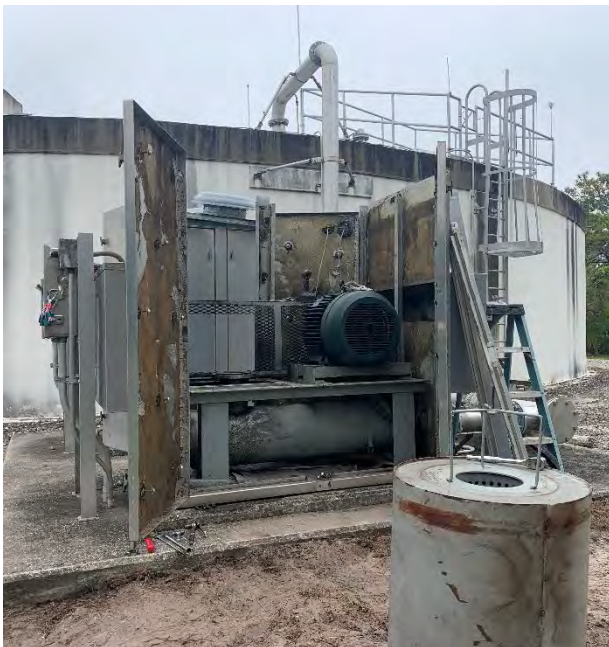
Biosolids Storage Tank – Process Air Blower Replacement
