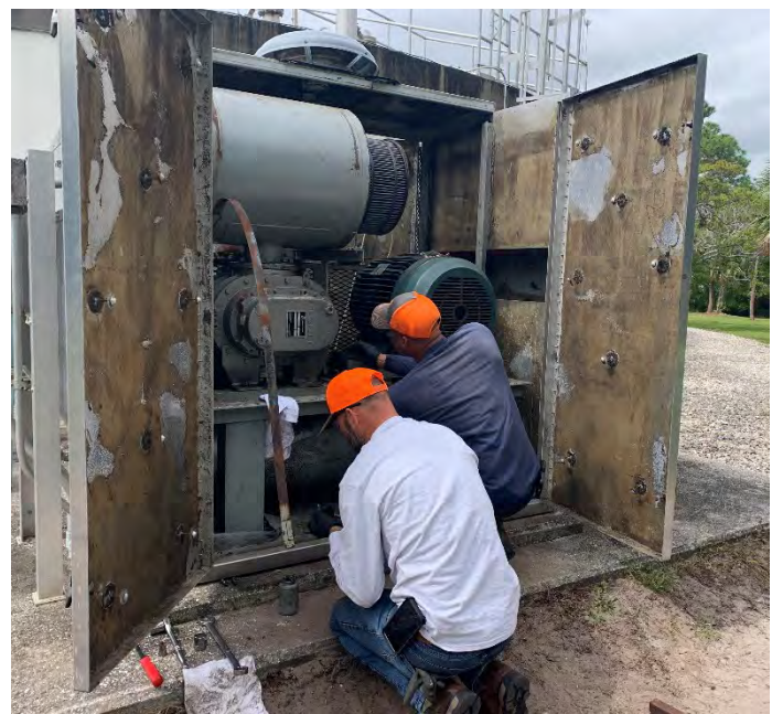
Biosolids Storage Tank – Process Air Blower Replacement
