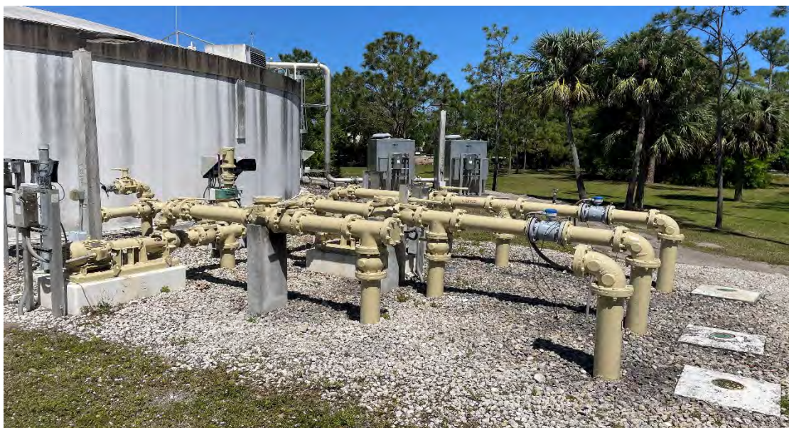
Biosolids Transfer Pumps and Piping
