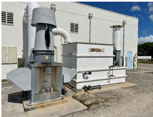
Chlorine Building Air Scrubber Unit
