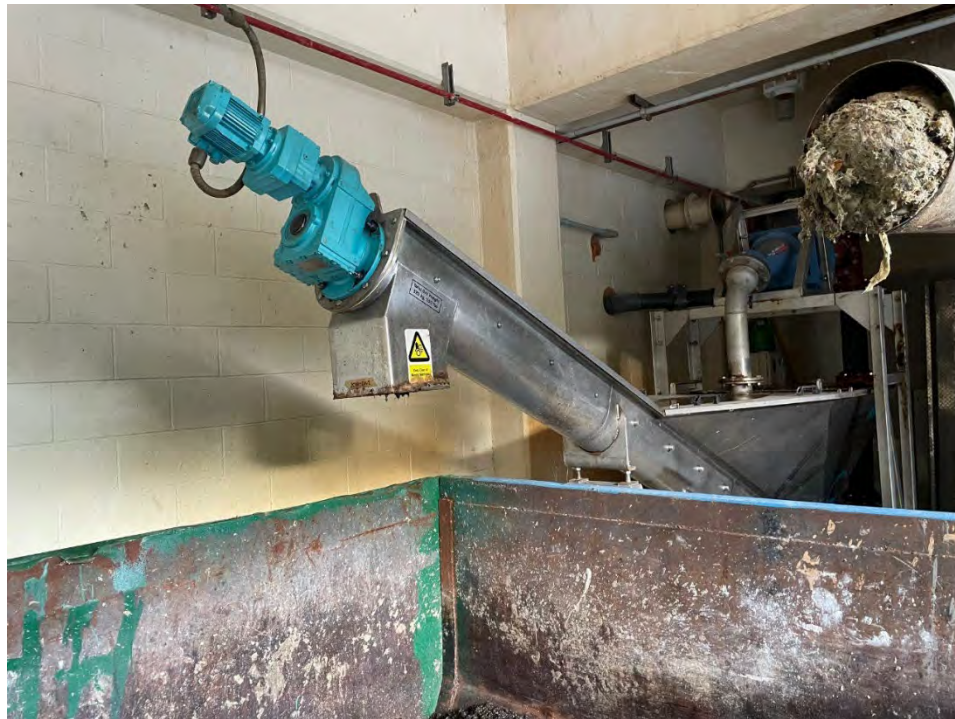
Grit Classifier – Gear Reducer and Motor Replacement
