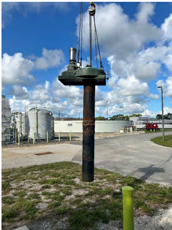
Grit Drive and Tube Assembly - Pre and Post Repair
