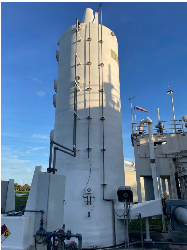
Headworks Odor Control System – H_2S Analyzer
