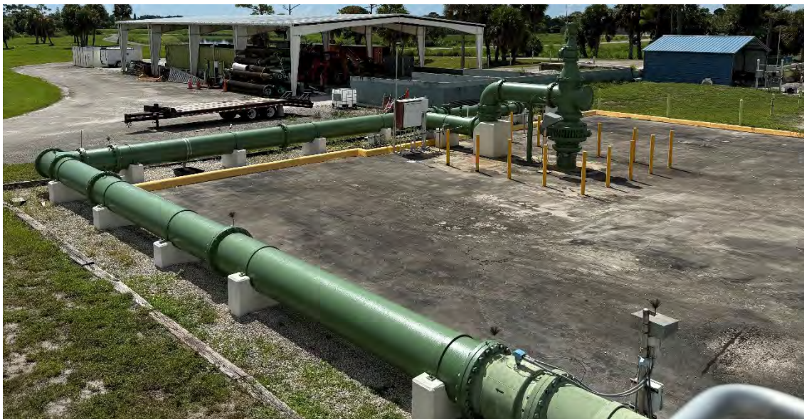
Deep Injection Wellhead and Piping
