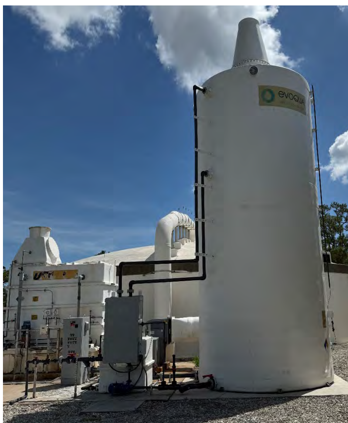
Biotrickling Odor Control System Installation
