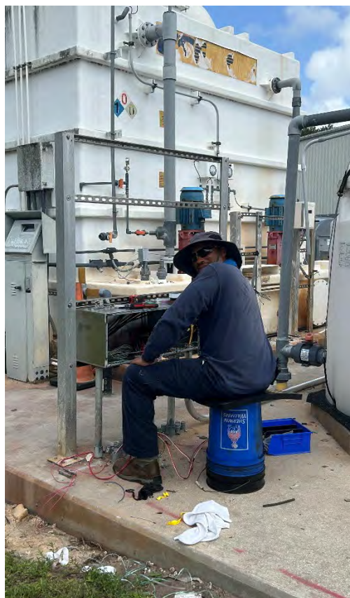
Installation of Biotrickling Odor System Utilities
