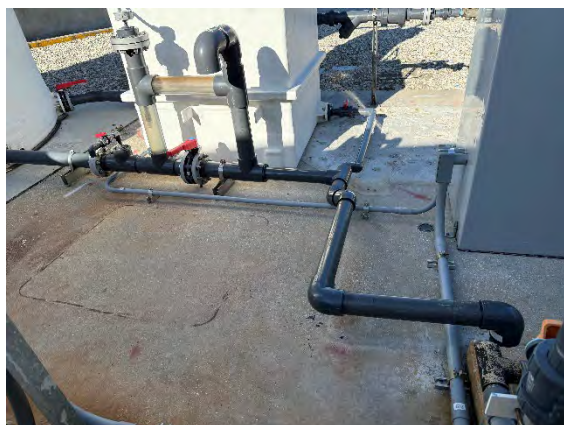
Installation of Biotrickling Odor System Utilities
