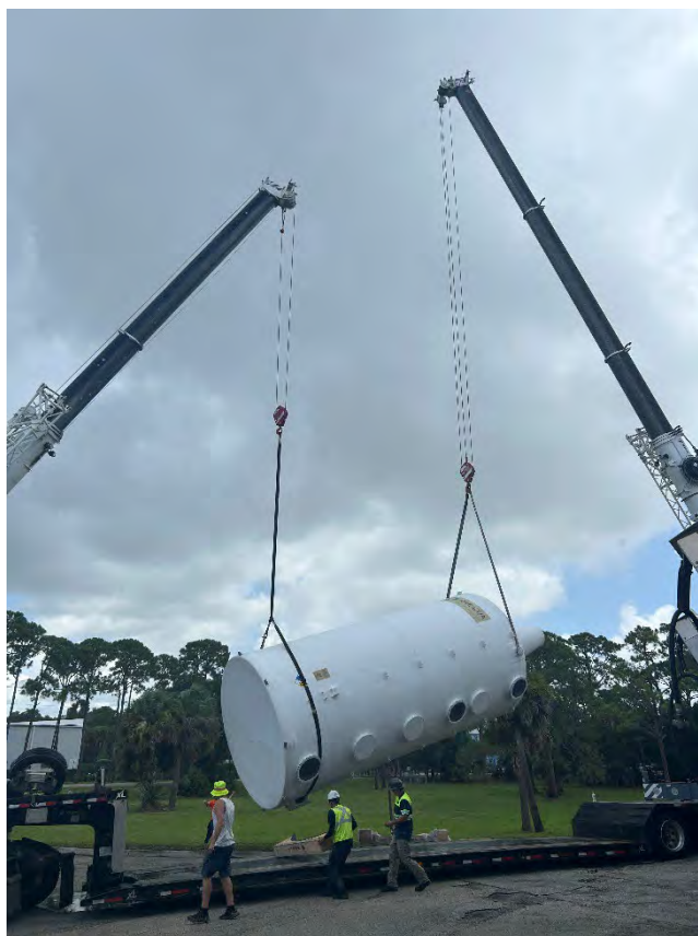
Biotrickling Odor Control System Installation
