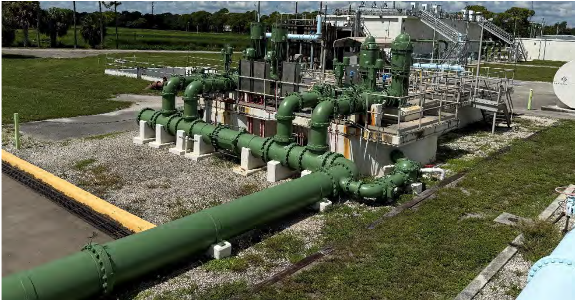
Injection Well Pump Station and Piping
