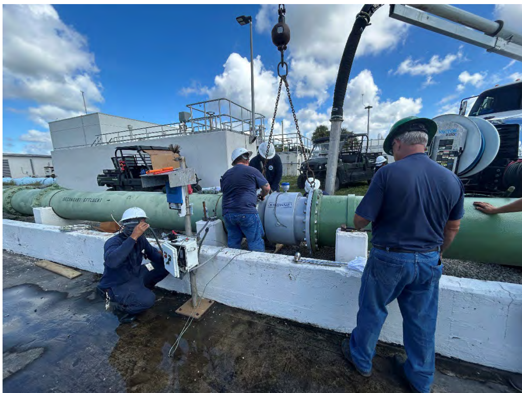
Injection Well Flow Meter Tube and Transmitter Replacement
