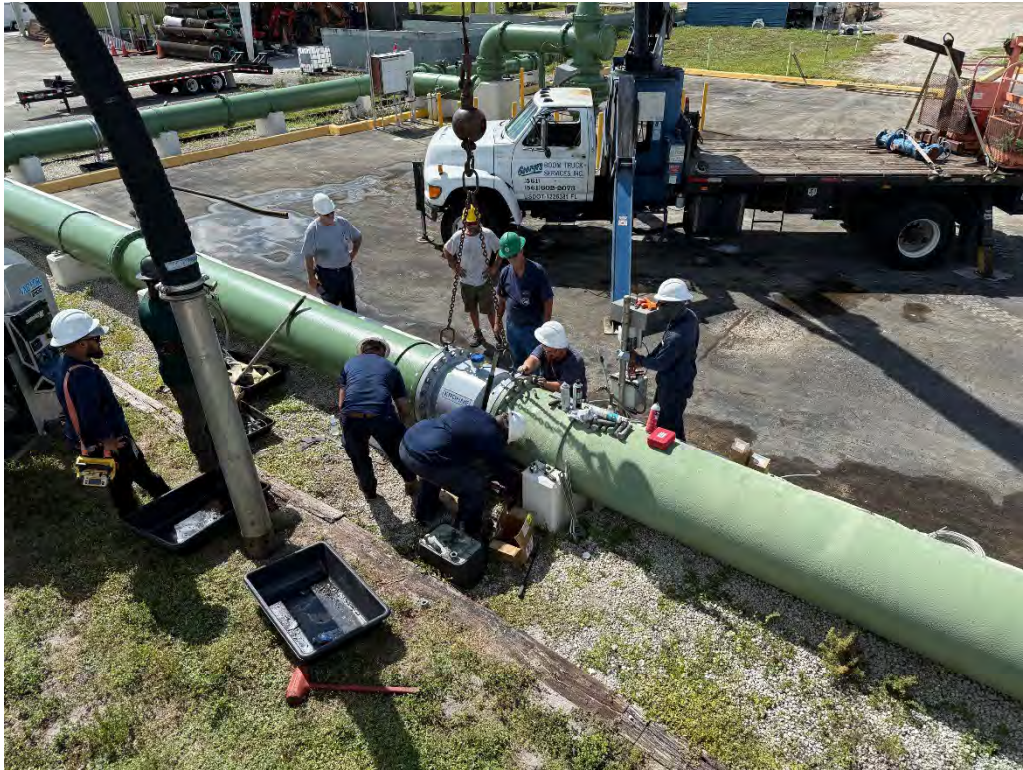
Injection Well Flow Meter Tube Replacement
