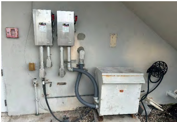
Ops Control Bldg. – Main Disconnect
