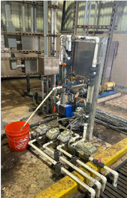
Existing and Replacement Polymer Mixing and Feed Units
