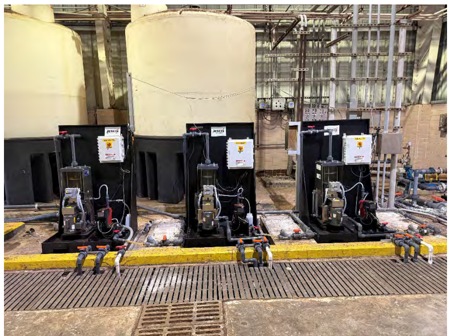
Existing and Replacement Polymer Mixing and Feed Units
