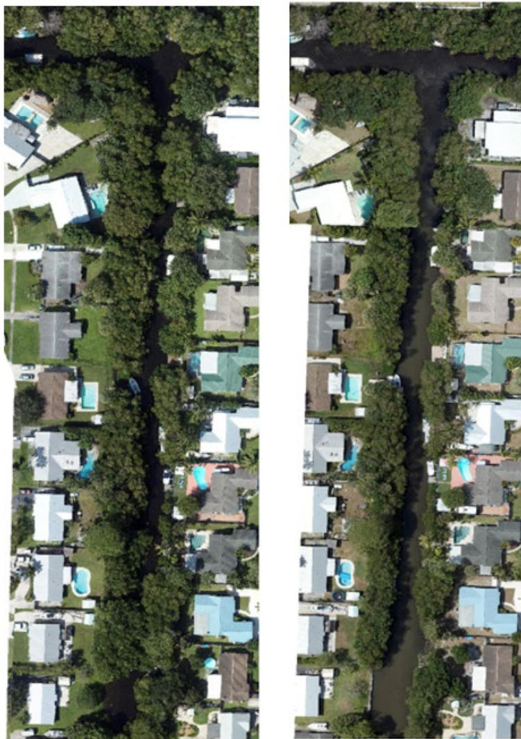
Figure S13. Section of Jones Creek between Pawnee Street to the west and Pennock Lane to the east. Drone imagery taken before trimming (left) and after trimming (right).
