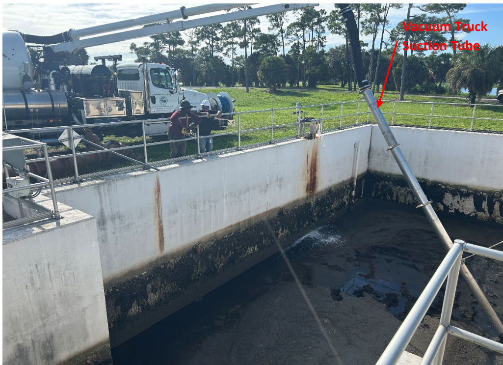
Filter Backwash Basin – Cleaning In-Process
