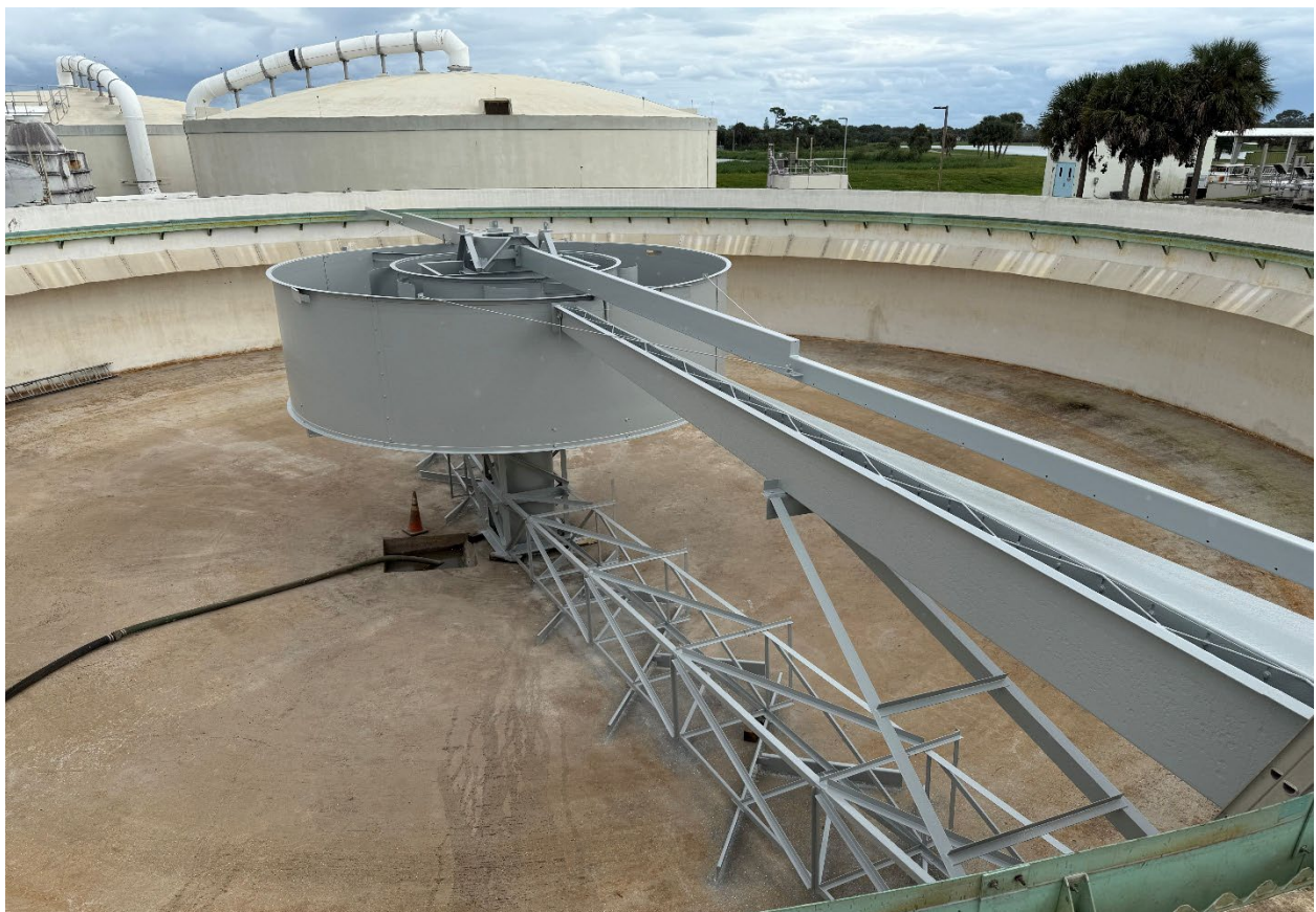
Clarifier No. 4 – Post Surface Preparation and Coating
