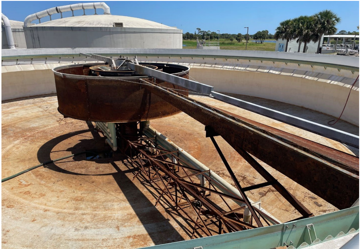
Clarifier No. 4 – Pre Surface Preparation and Coating
