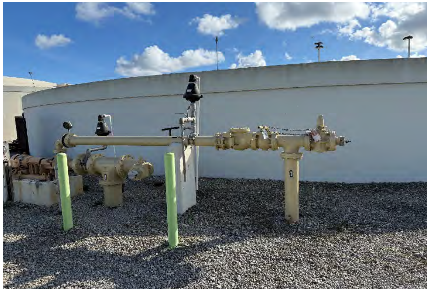
WAS Pump No. 4 – Check Valve Replacement
