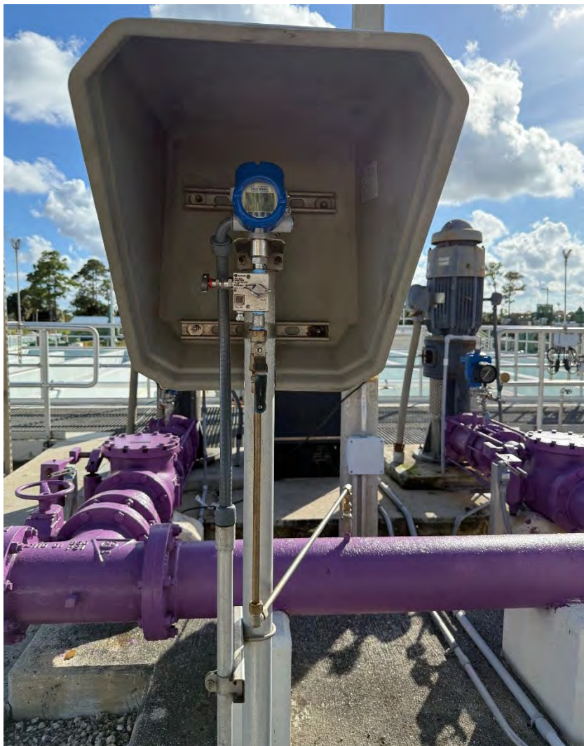
Non-Potable Water Distribution System – Pressure Transmitter
