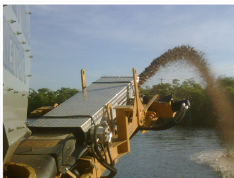
The Sand Shooter at work capping muck sediments
