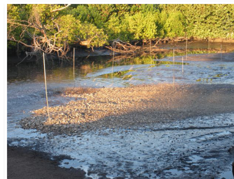
Fossil Shell placed over 7' of muck sediments
