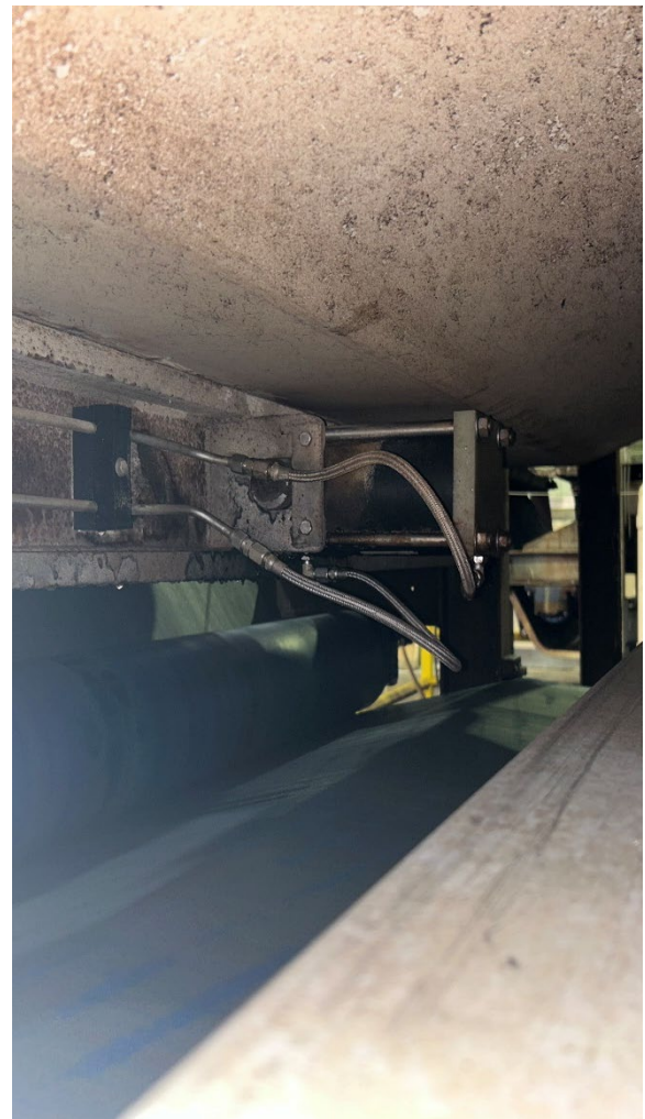
Belt Filter Press No. 1 – Hydraulic Cylinder Replacement
