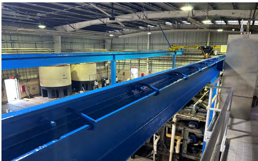
Solids Dewatering Facility OH Crane – Post-Work
