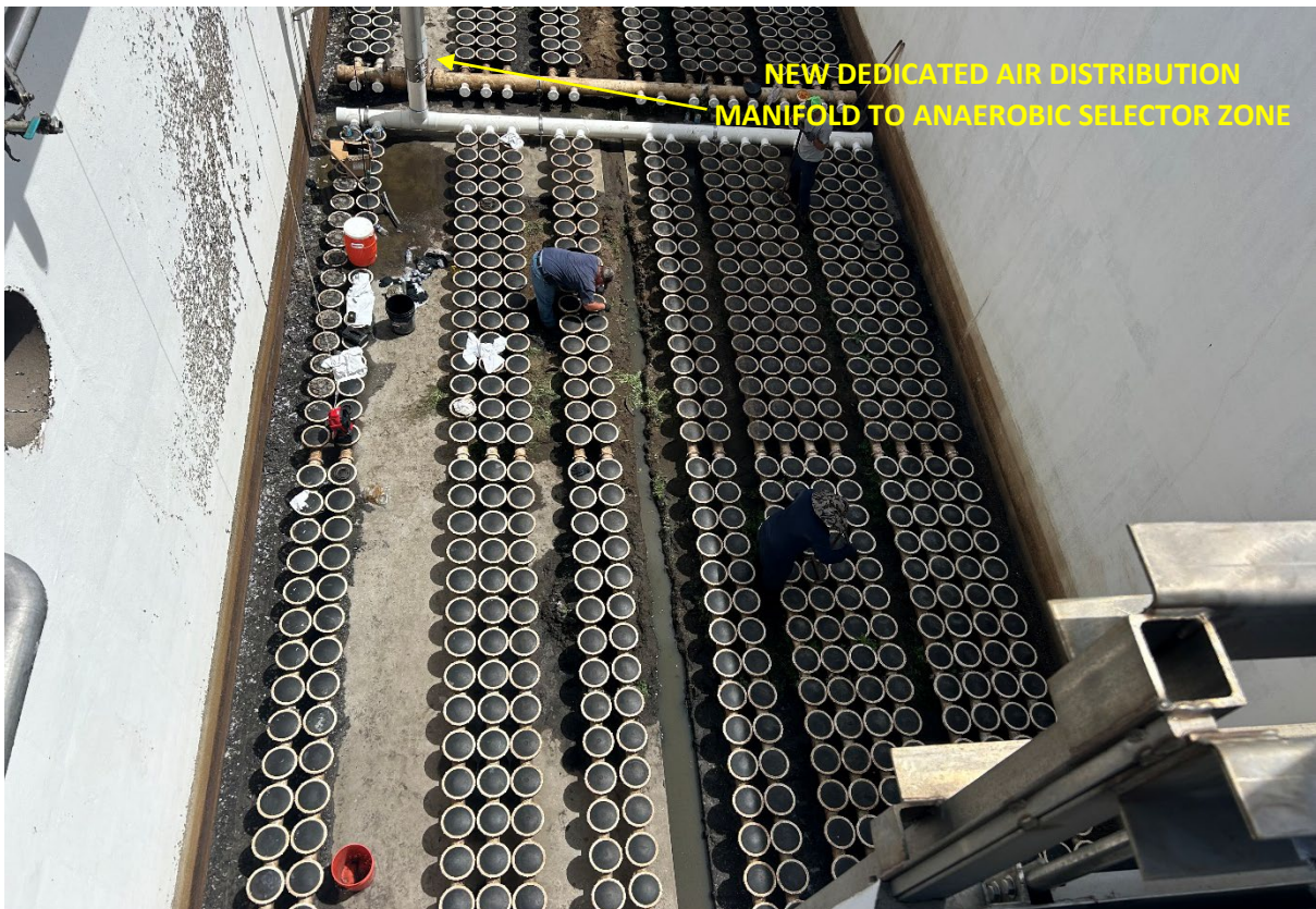
Aeration Basin No. 1 – Process Air Piping Modification
