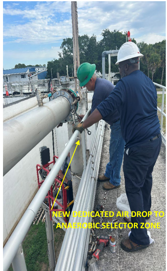
AB-3 Diffused Aeration Upgrades
