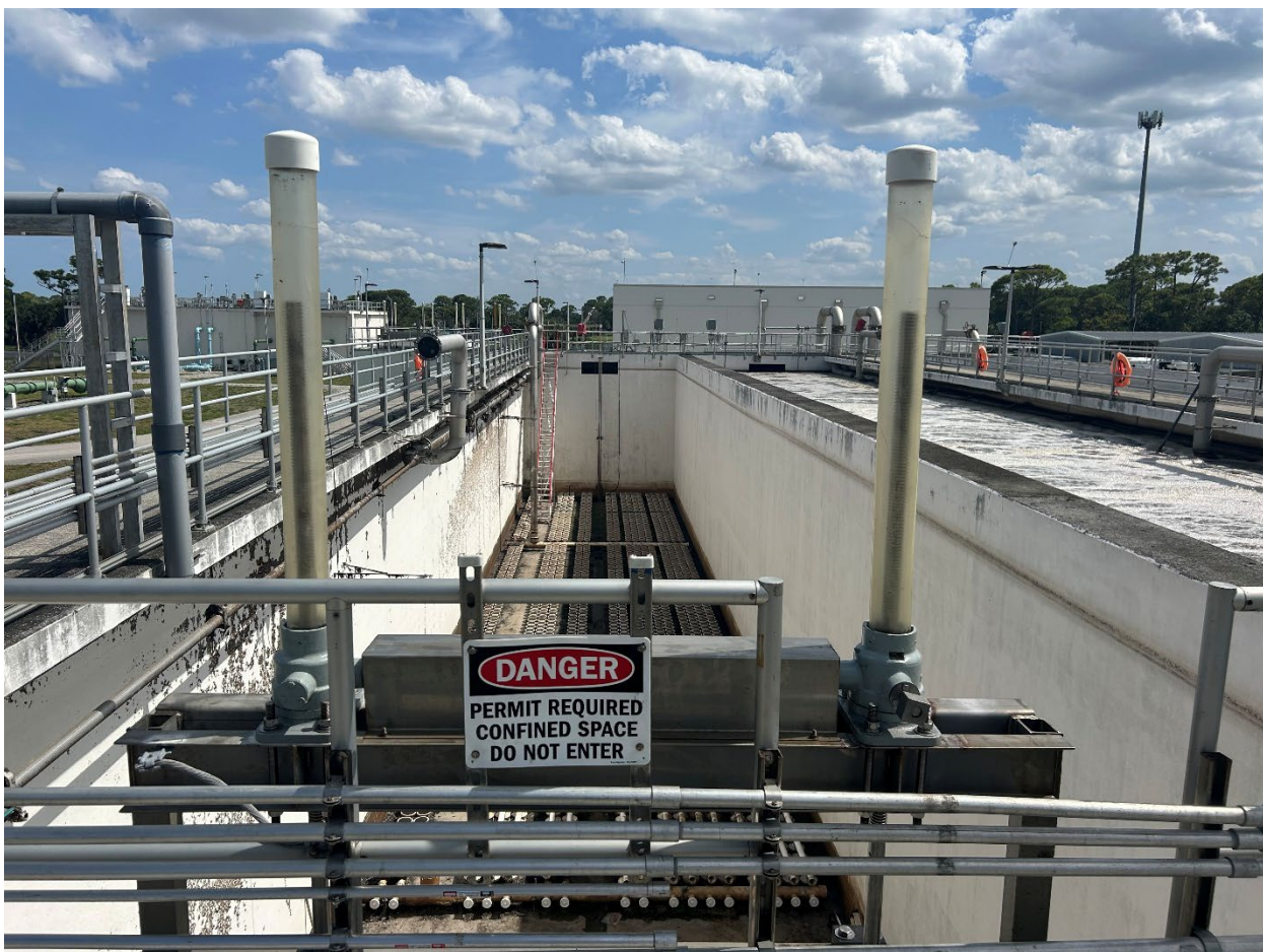
Aeration Basin No. 1 - New Manually Operated Gate Operator
