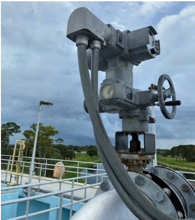
Backwash Air Control Valve Maintenance
