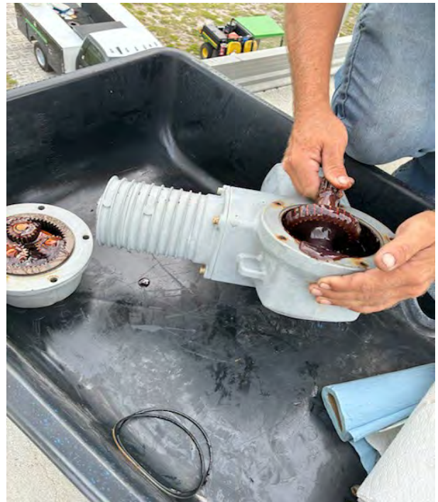
Backwash Air Control Valve Maintenance
