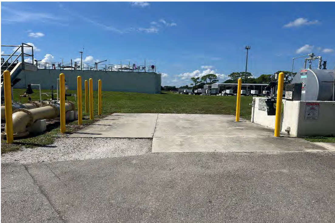
Vehicle Protection Bollard Enhancements
