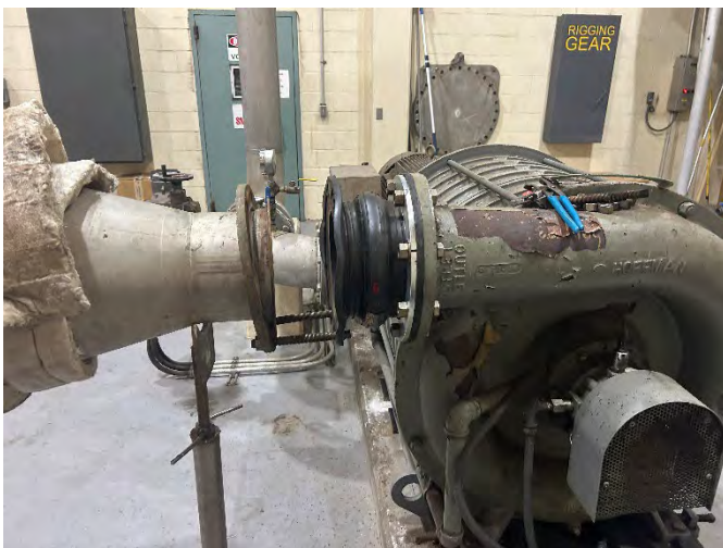
Process Air Blower – Check Valve Replacement
