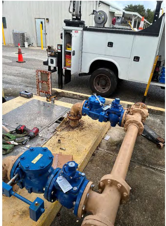
Plant Lift Station No. 2 – Valve Replacement
