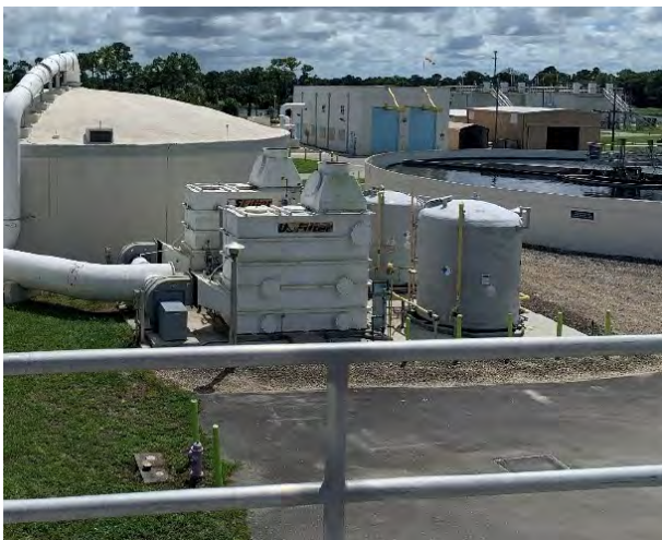
EQ Odor Control System – Pre-Demolition
