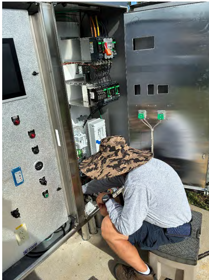
Plant Lift Station No. 1 – Pump No. 1 Temporary Soft Start Installation
