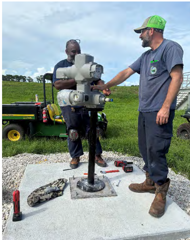
Nano Concentrate Isolation Valve – Motor Actuator Improvements
