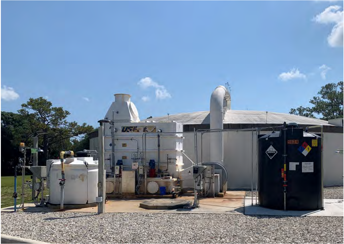
SST Odor Control System – Pre-Demolition
