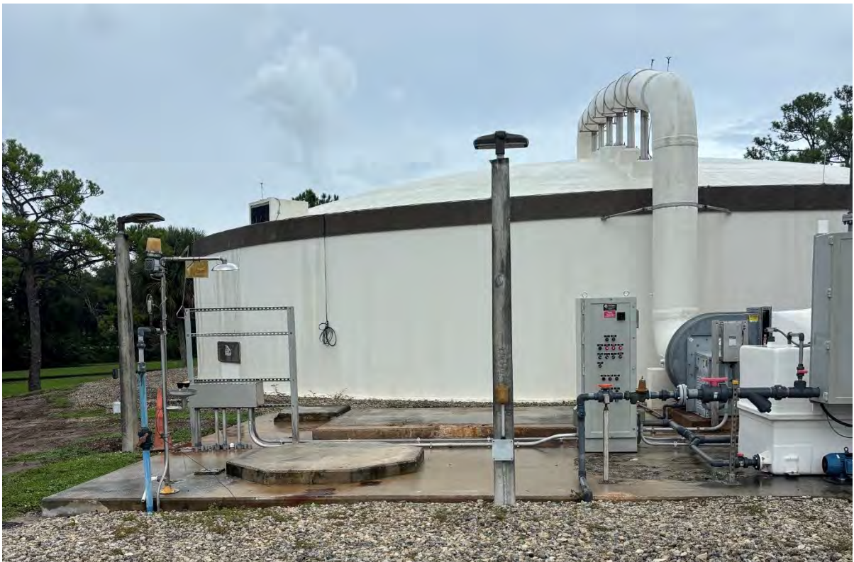
SST Odor Control System – Post-Demolition
