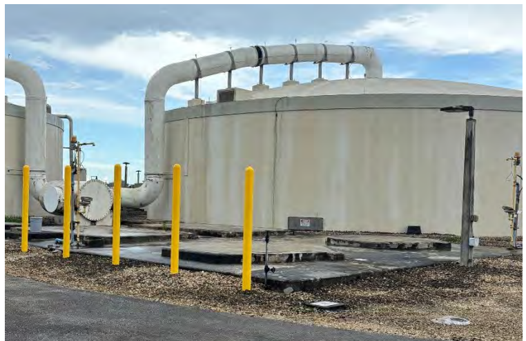
EQ Odor Control System – Post-Demolition
